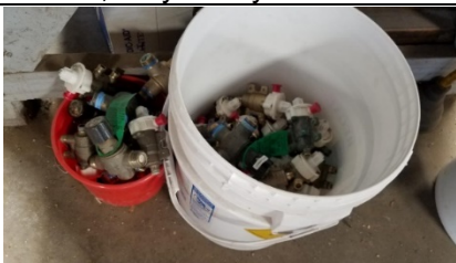
Bucket of failed mixing valves
